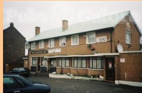
Maltese Cat , Roehampton, south-west London. The pub closed in October 2004 and was later demolished for flats.
